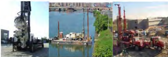
Sonic Drills East River Project Shaker School Project
